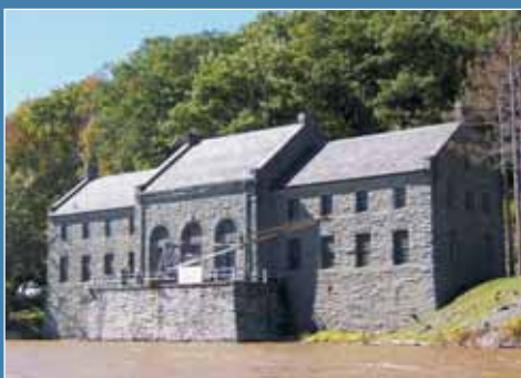
Shandaken Intake Building, Schoharie Reservoir
