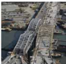
NYSOT, Willis Avenue Bridge
