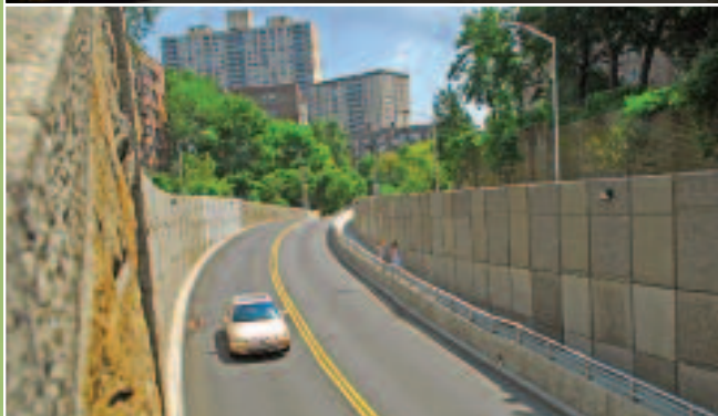
THE KAPOCK STREET RETAINING WALL Structural Systems Category
