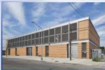
Amtrak East River Tunnel Ventilation Building, Long Island City, NY
