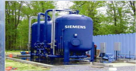
Construction of the Granular Activated Carbon Treatment System (GAC)
