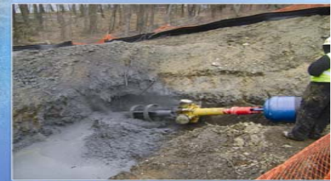
Directional Drilling - Final 36" Ream
