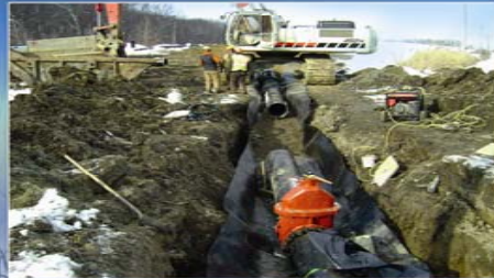
Pipeline Construction Over a Closed Landfill
